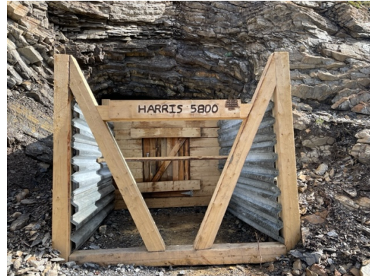
Photo 14 – 5800 Level Harris Vein Adit After
