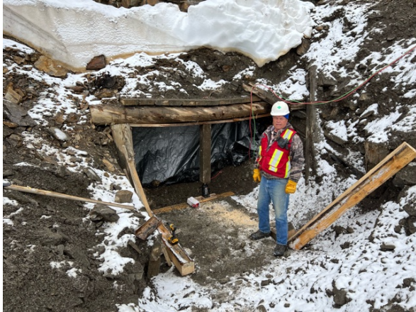
Photo 7- Final door installed on Davis Keays 6400 level.
