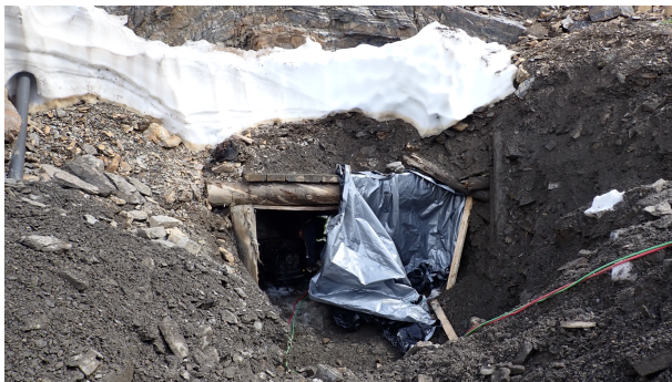
Photo 3 – Cleaning 6400 level adit
