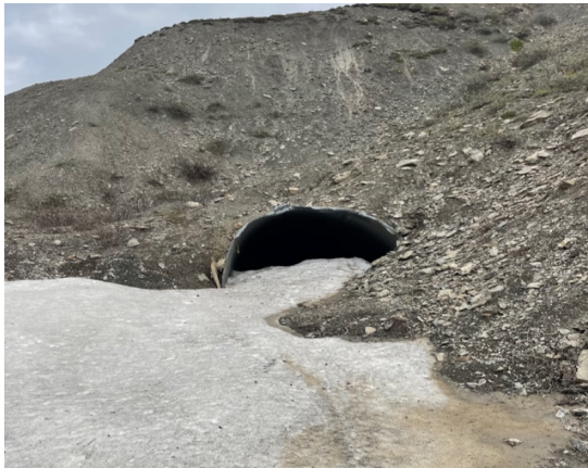
Photo 15 – 5200 Level Magnum Mine before
