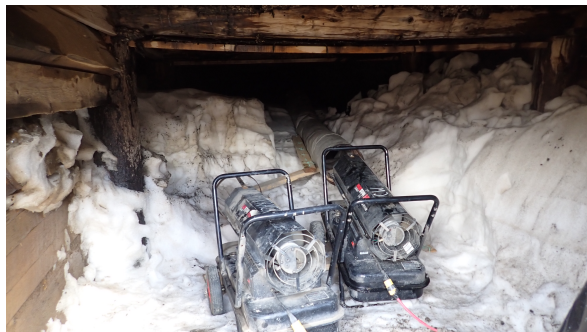
Photo 4 – Heaters in Entrance
