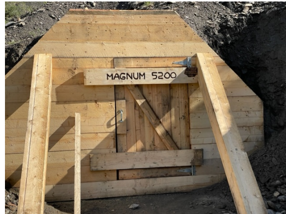
Photo 16 – 5200 level magnum Mine After
