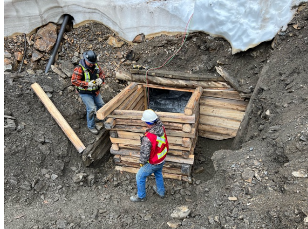
Photo 6 – Tower Being Constructed
