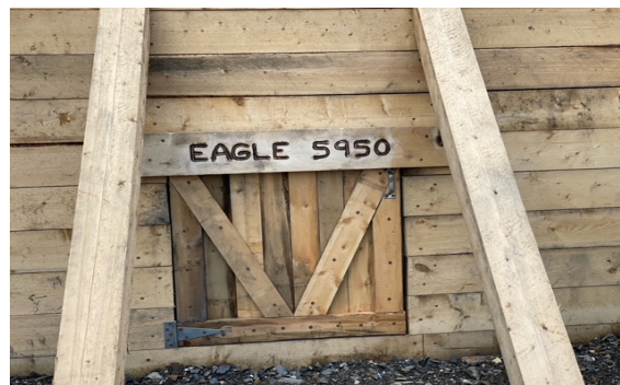
Photo 12 - Final door installed on Davis Keays 5950 level.
