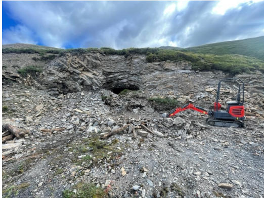
Photo 13 – 5800 Level Harris Vein Adit Before
